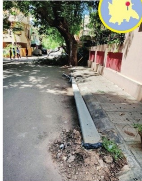
An electrical pole has fallen again at 12th cross, RT Nagar 1st block.
