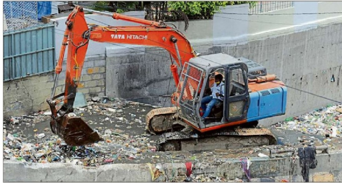
Cleaning a clogged stormwater drain. DH FILE
